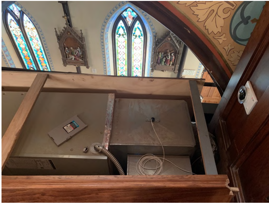
Figure 1: AHU-3 in loft area, not functional
