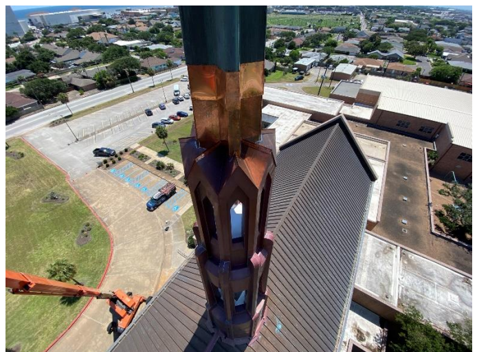
Photo12: Completed Copper on North Side of Needle
