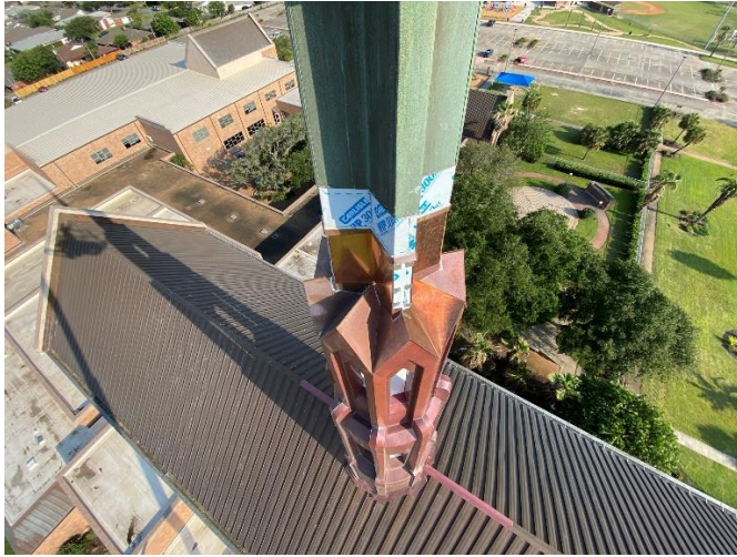
Photo09: New Copper Panels Installed on Base of Needle
