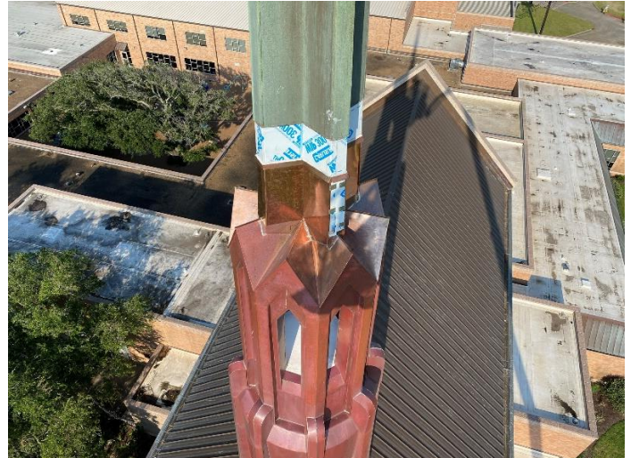
Photo06: New Copper Panels Installed on Base of Needle
