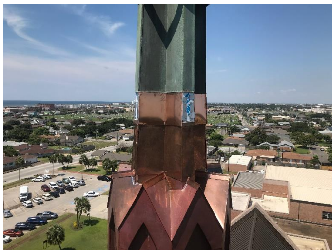
Photo11: New Copper and Stainless Steel Clips Installed
