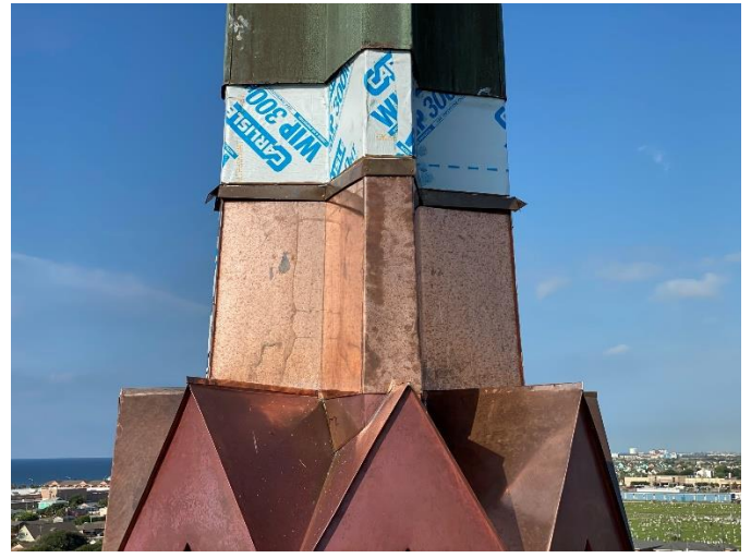
Photo08: New Copper Panels Installed on Base of Needle
