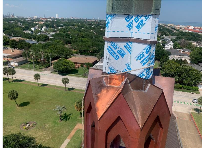
Photo02: Copper Flashing Installed on Steel Structure Edge
