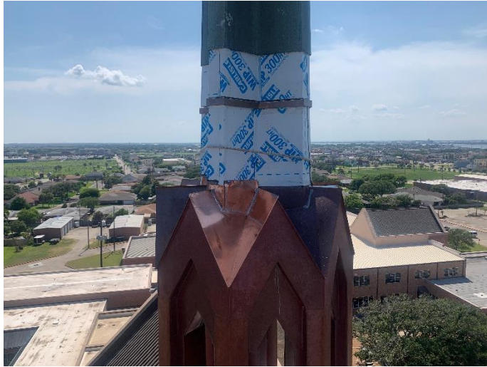
Photo01: Copper Flashing Installed on Steel Structure Edge
