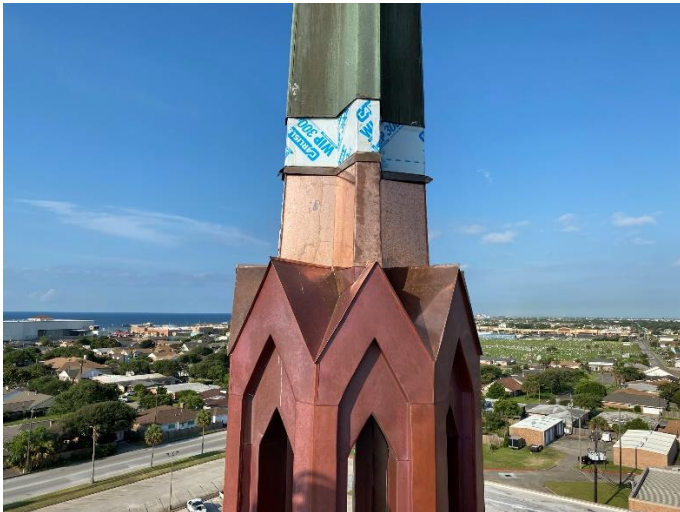
Photo07: New Copper Panels Installed on Base of Needle
