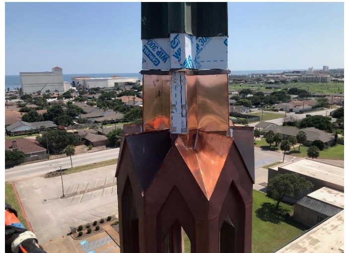
Photo04: New Copper Panels Installed on Base of Needle
