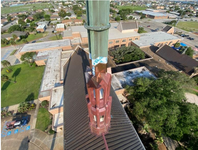
Photo05: New Copper Panels Installed on Base of Needle
