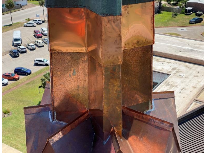
Photo13: Completed Copper View of Needle
