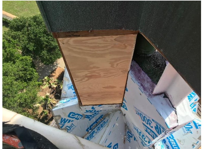
Photo10: New Plywood Piece Installed Adjacent to Newly Waterproofed Plywood and Boards
