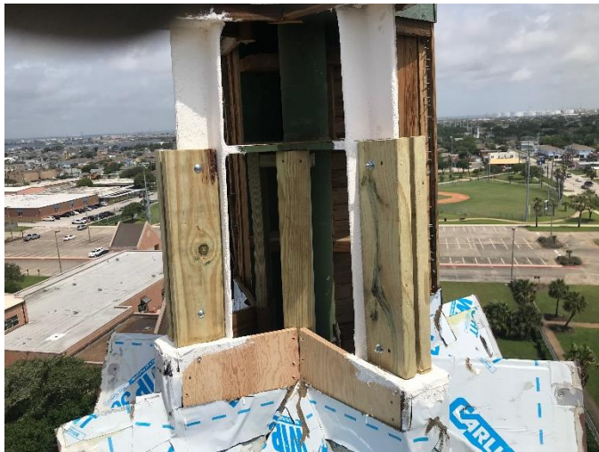
Photo07: New Boards Fastened to the Steel Structure
