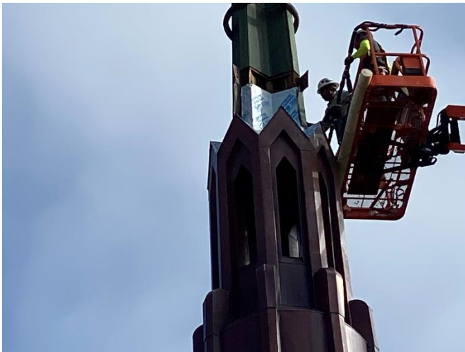
Photo01: Workers Removing Temporary Waterproofing and Copper Cladding of Spire
