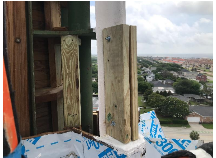
Photo06: New Wooden Boards are Installed on the Steel Structure
