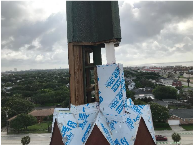
Photo09: Waterproofing Installed on New Plywood and Boards
