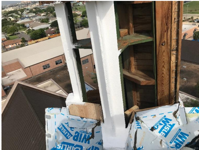
Photo05: Steel Structure Coated in Liquid Waterproofing
