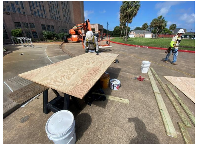
Photo04: Marine Grade Plywood Measured and Cut for Installation
