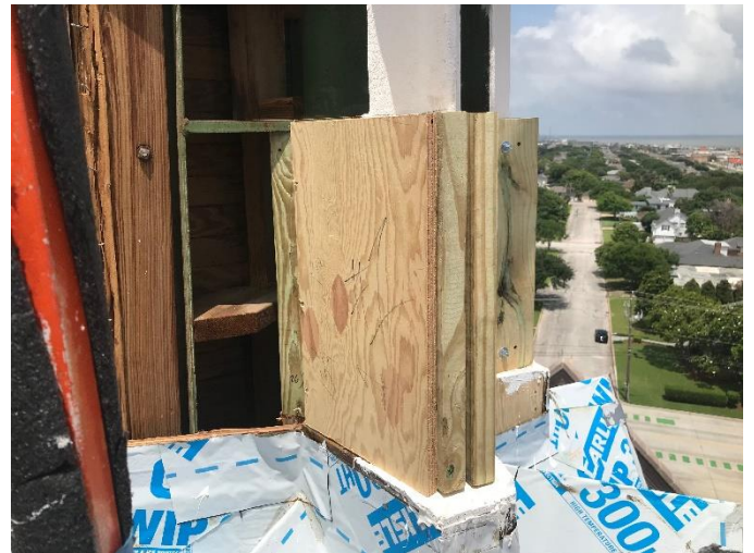
Photo08: Plywood Fastened to Boards and Steel Structure
