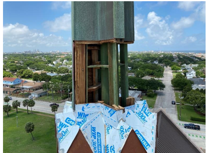
Photo02: Old Wooden Boards are Removed
