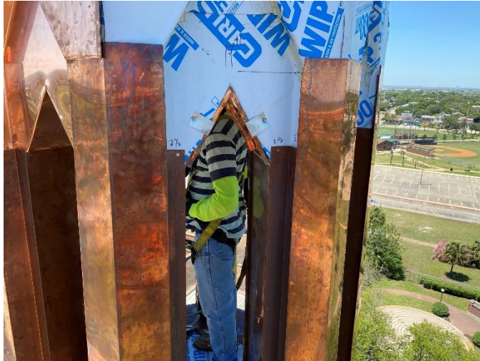
Photo13: Triangular Piece Installed at Soffit of Crown in Upper Belfry
