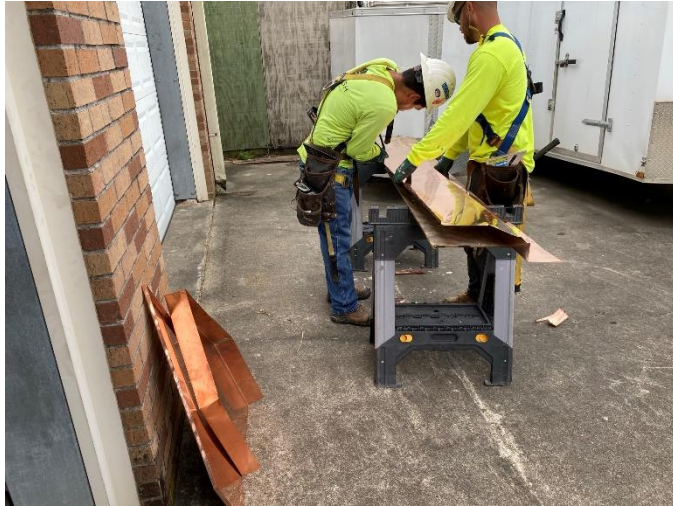
Photo01: Copper Pieces are Fabricated on Ground
