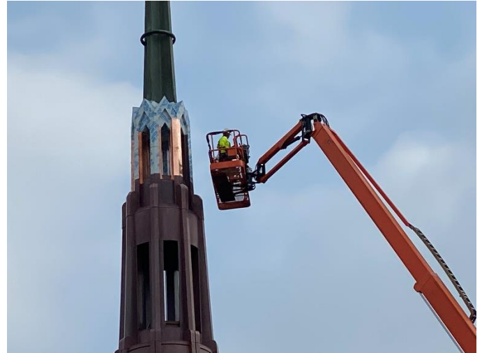
Photo06: First Outer Copper Piece Installed on Strut
