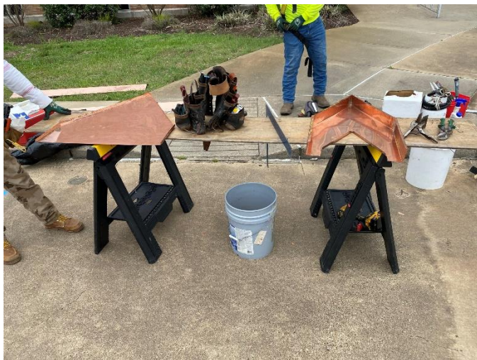
Photo07: Copper Face Pieces for the Crown of the Upper Tier are Fabricated
