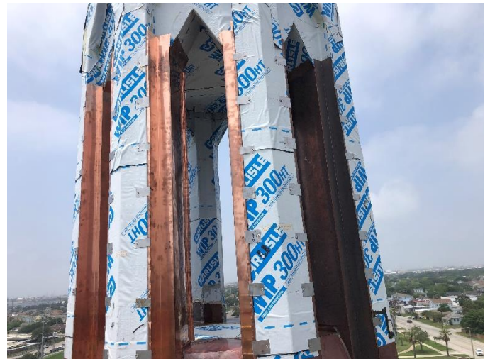
Photo04: Inner Strut Pieces Fastened with Stainless Steel Clips and Screws
