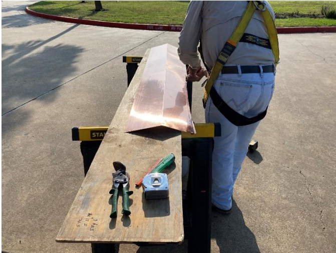
Photo09: Outer Facing Strut Pieces are Fabricated on the Ground
