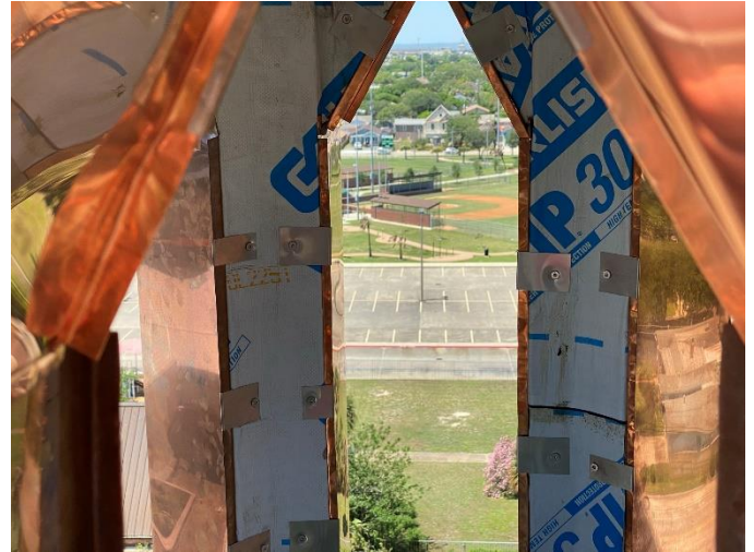
Photo14: Soffit Pieces and Inner Side of Upper Belfry
