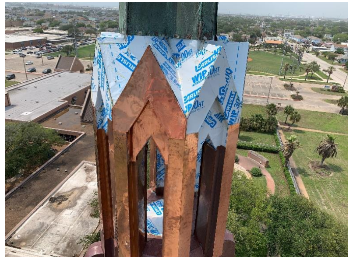
Photo12: The First Copper Face Piece for the Crown of the Upper Tier is Installed
