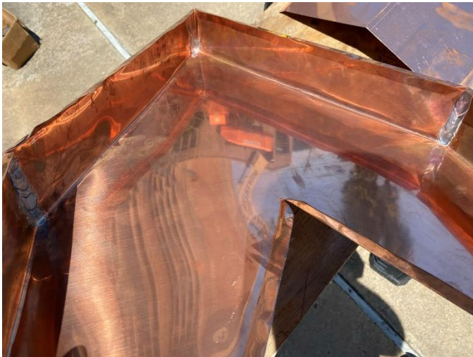
Photo11: Copper Face Plate for the Crown of the Upper Tier is Soldered at the Joints
