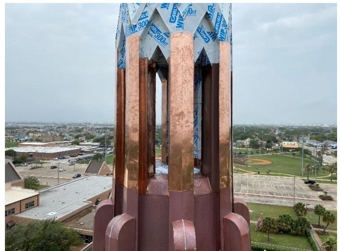
Photo08: Outer Copper Pieces after Installation
