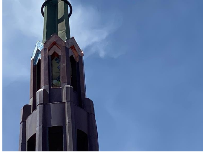
Photo18: Copper Face Plates Installed at the Crown of the Upper Tier
