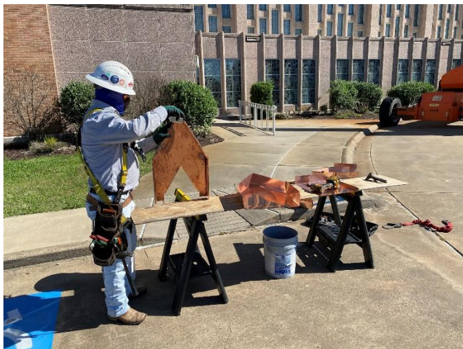
Photo15: Copper Face Pieces for the Crown of the Upper Tier are Fabricated on the Ground
