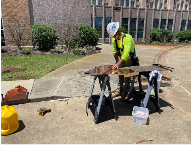
Photo17: Copper Face Pieces for the Crown of the Upper Tier are Fabricated on the Ground
