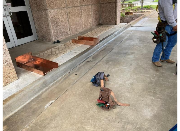
Photo06: Copper Panel Pieces are Fabricated
