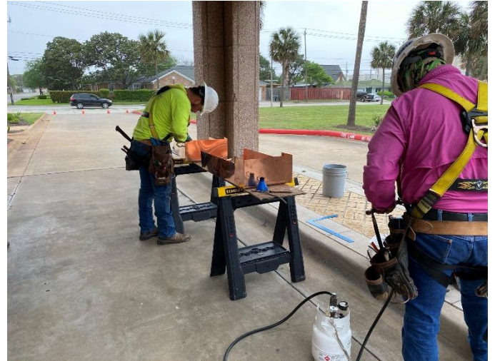
Photo10: Copper Panel Pieces are Fabricated
