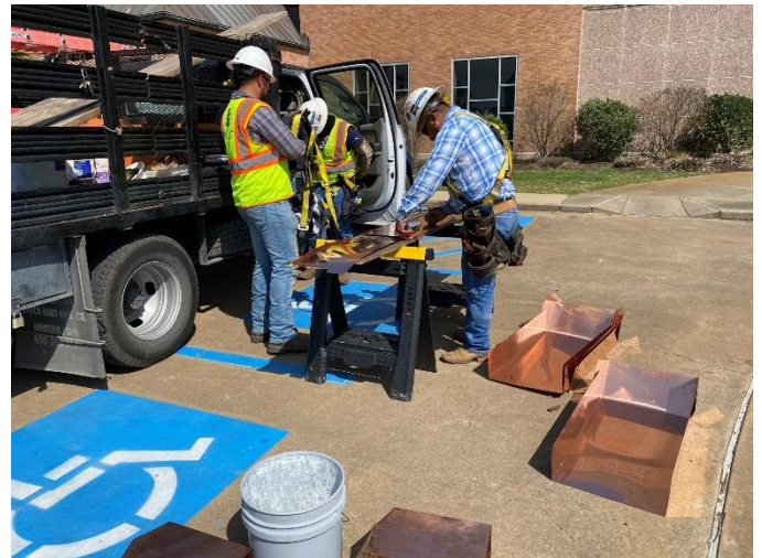
Photo04: Copper Pieces are Fabricated on Ground
