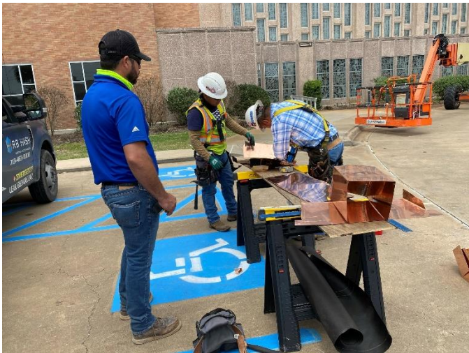
Photo03: Copper Pieces are Fabricated on Ground
