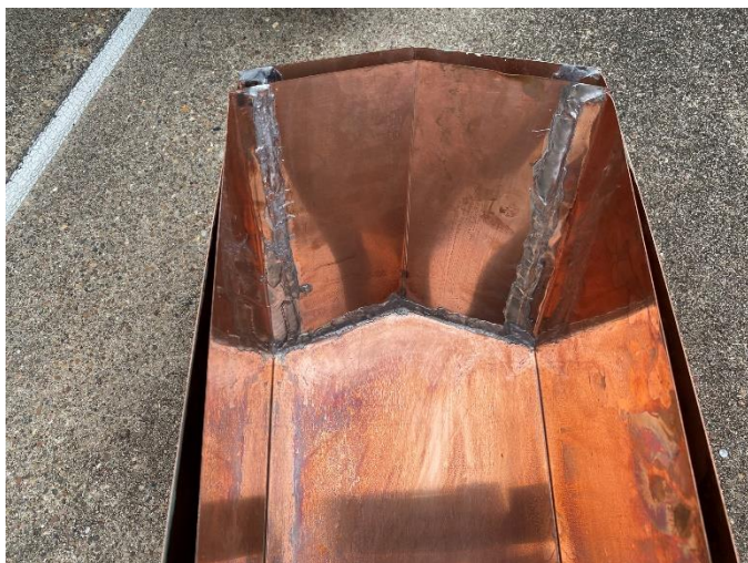
Photo13: Cap Pieces Have Been Soldered at Seams
