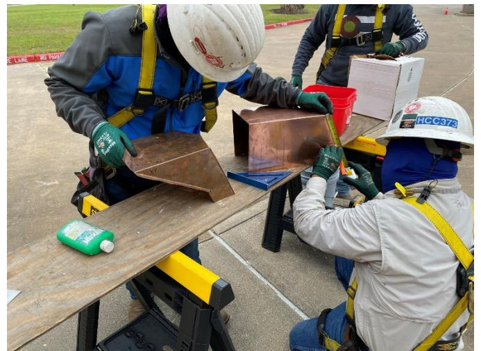
Photo12: Caps for the Long Struts of the Middle Tier are Fabricated
