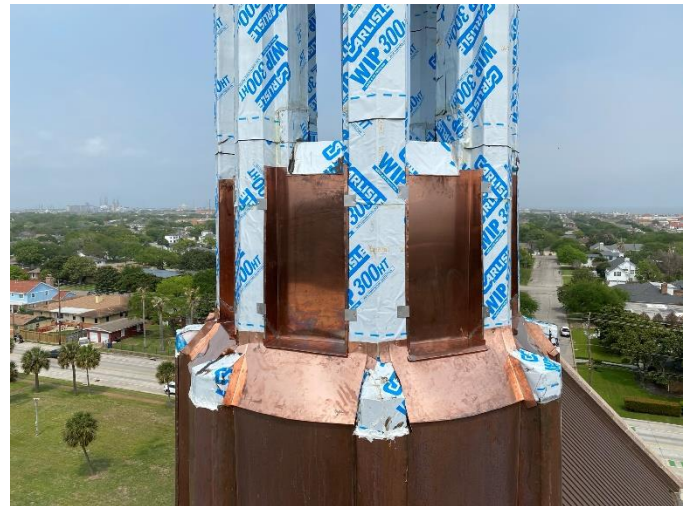
Photo08: Copper Panel Pieces Installed on Upper Tier of Steeple
