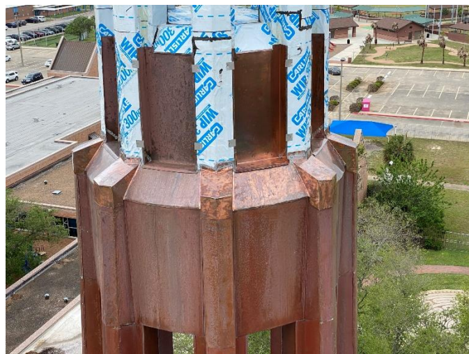
Photo14: Cap Pieces Installed at Top of Mid-Tier Struts
