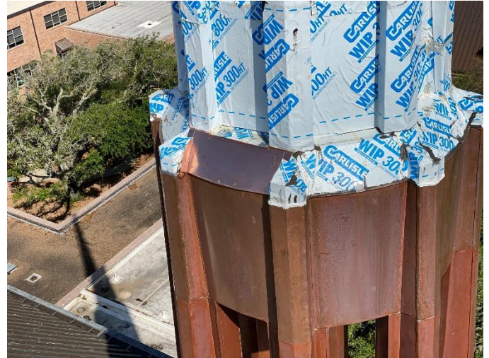
Photo02: First Copper Piece Installed on Upper Tier of Steeple
