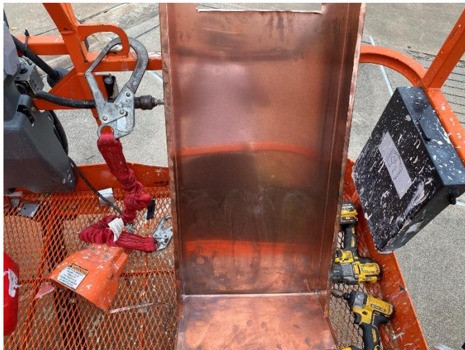
Photo07: Copper Panel Piece Prior to Installation
