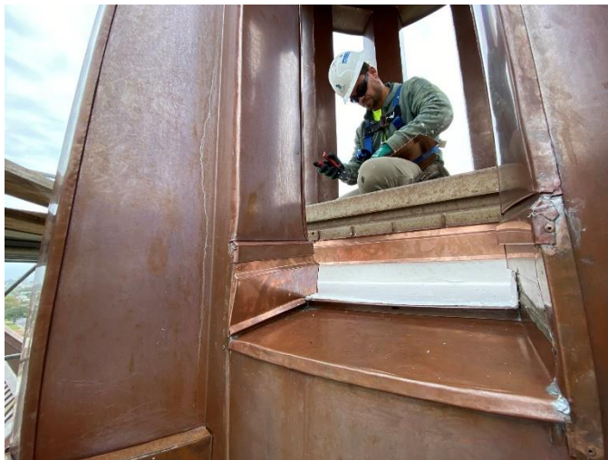
Photo09: Copper Flashing Installed on the Side of the Base of the Mid-Tier Struts
