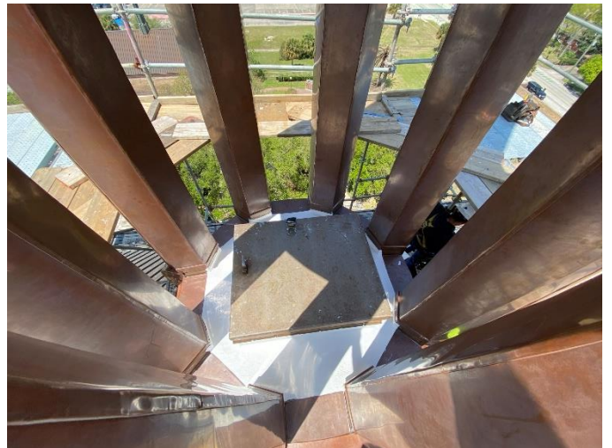
Photo04: Parapro Flashing Resin Applied at Floor of Belfry
