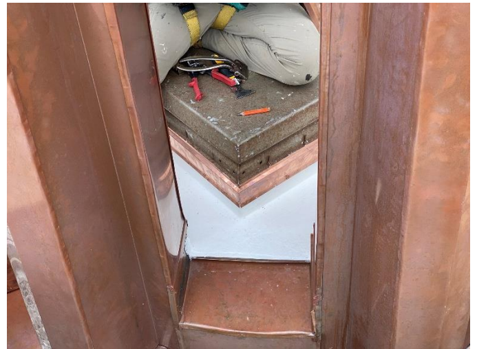
Photo08: Copper Flashing is Installed Around Hatch
