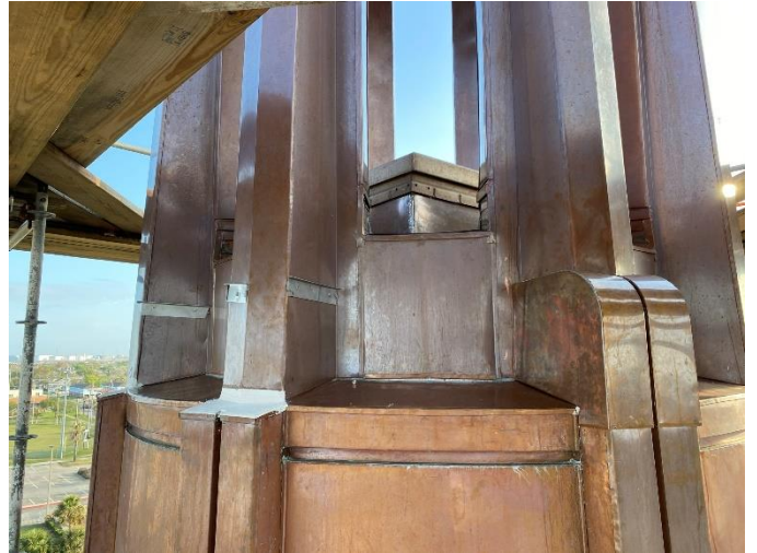
Photo02: Corner Edge Piece Installed, Top of Strut Coated in Liquid Flashing
