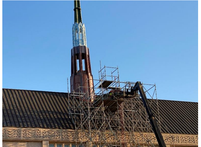
Photo16: Scaffold Materials are Loaded into the Fork Lift
