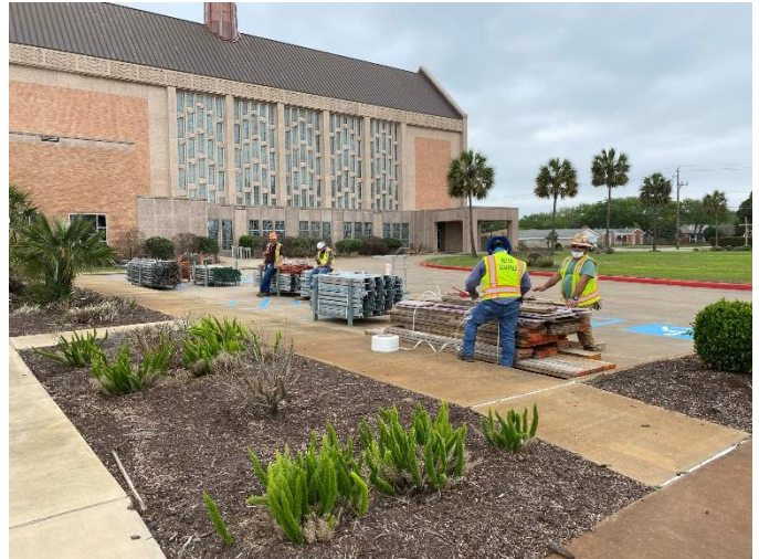
Photo20: Scaffold Materials are Tied Up for Pick Up
