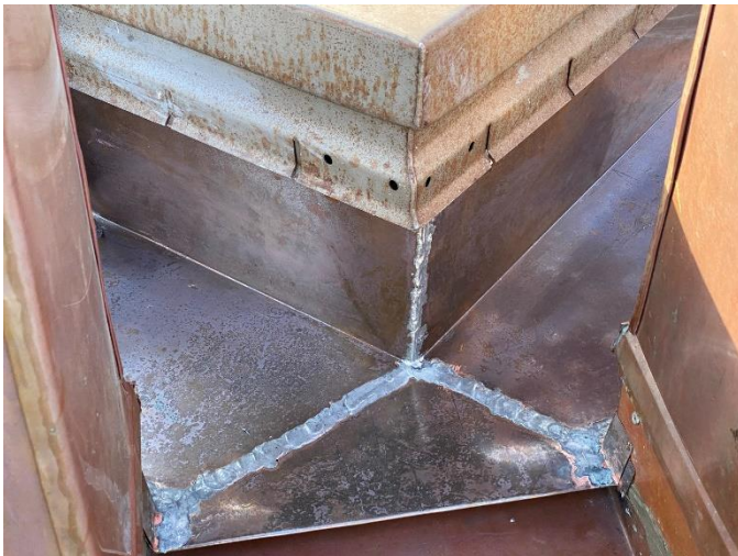
Photo03: Corner of Hatch Copper Soldered Together
