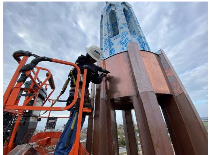
Photo10: Excess Copper Removed from Panel
