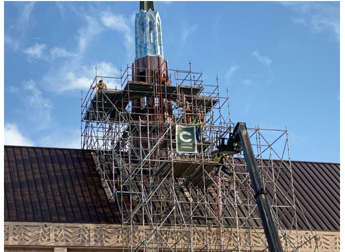
Photo12: Scaffolding is Disassembled
