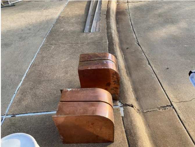
Photo01: Corner Edge Pieces Fabricated Before Installation
