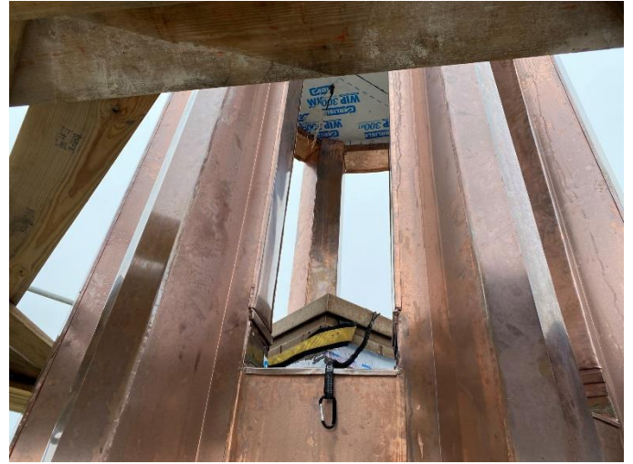
Photo10: Side Pieces and Ceiling Pieces are Installed
