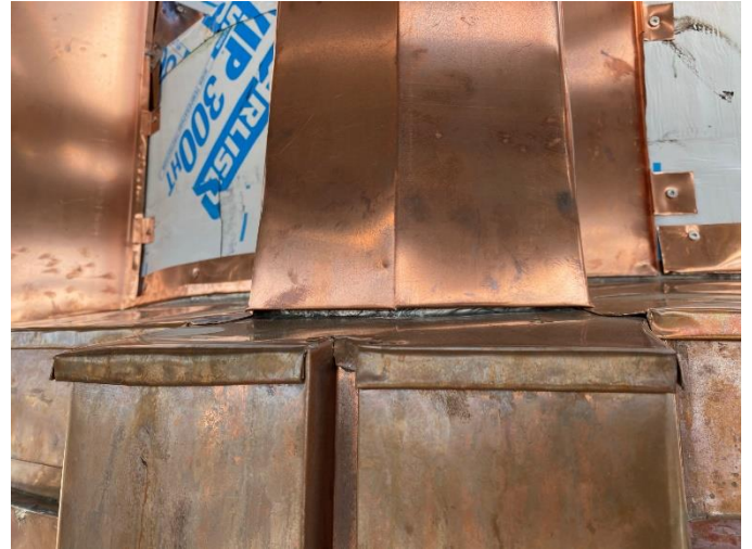
Photo02: Close-up of Soldered Area
