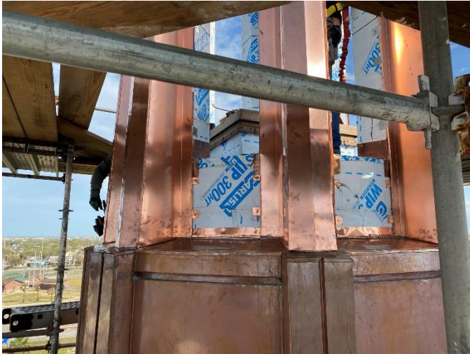
Photo01: Long Strut Pieces are Soldered to the Top of Base Tier
