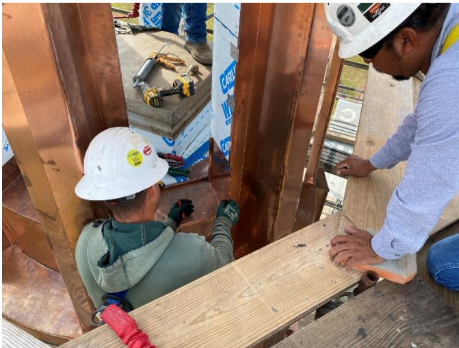
Photo03: Side Piece Fitted to Side of Strutt Piece
