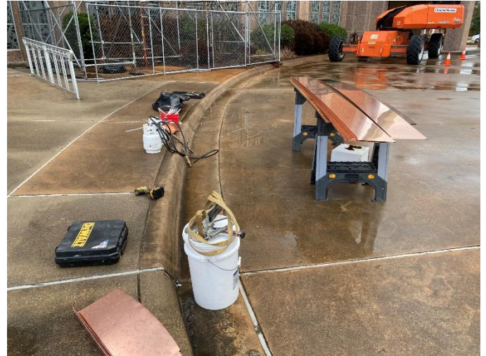
Photo06: New Copper Side Pieces Prepared for Installation
