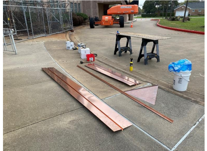
Photo14: Copper Pieces are Prepared for Installation
