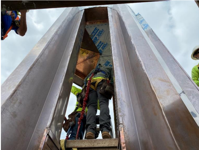
Photo17: Copper Ceiling Pieces are Installed at Hatch Access
