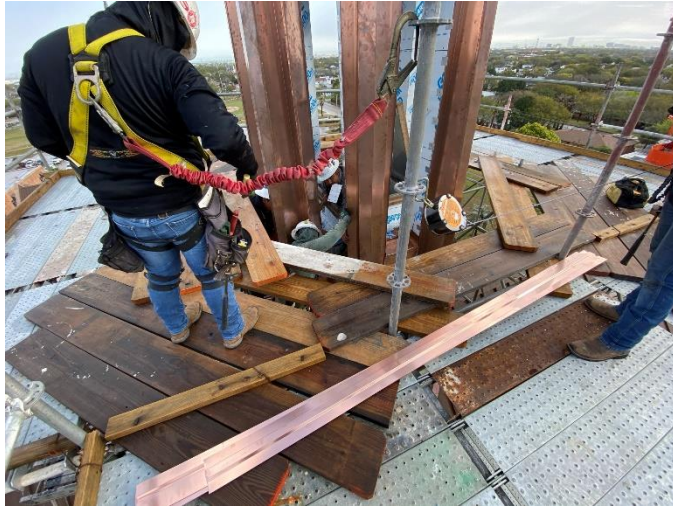
Photo05: Side Pieces Installed on Long Strut Pieces
