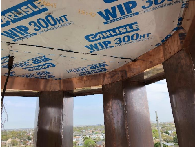
Photo13: Edge Metal Installed on the Interior Edge of Hatch Access
