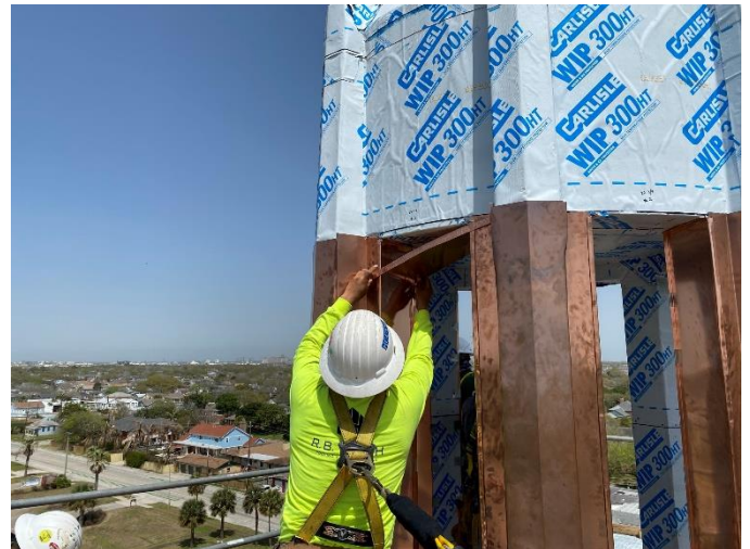
Photo08: Ceiling Pieces are Installed at Middle Tier
