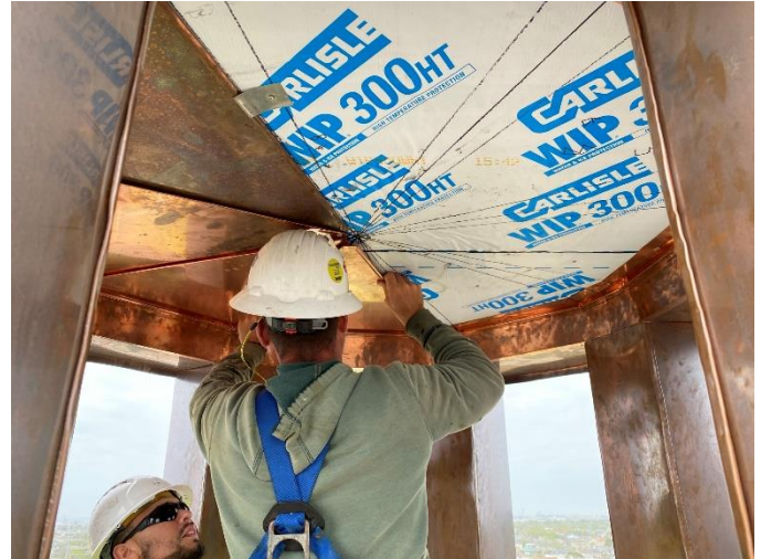
Photo18: Copper Ceiling Pieces are Installed at Hatch Access
