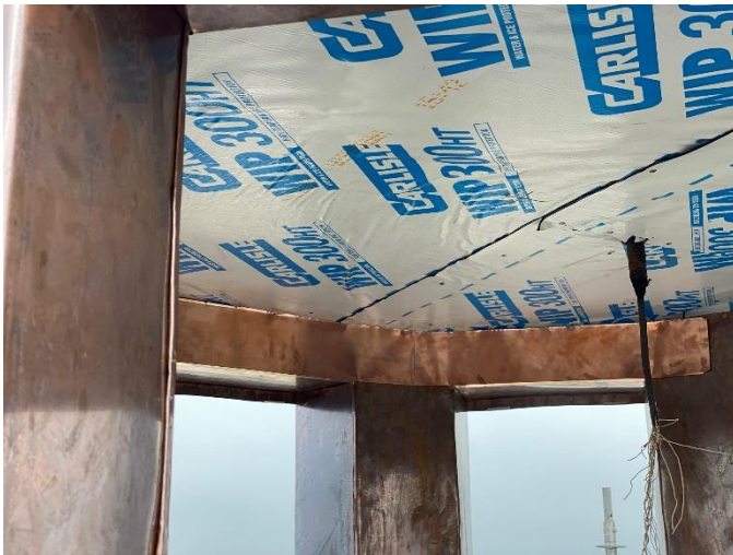
Photo11: Edge Metal Installed on the Interior Edge of Hatch Access
