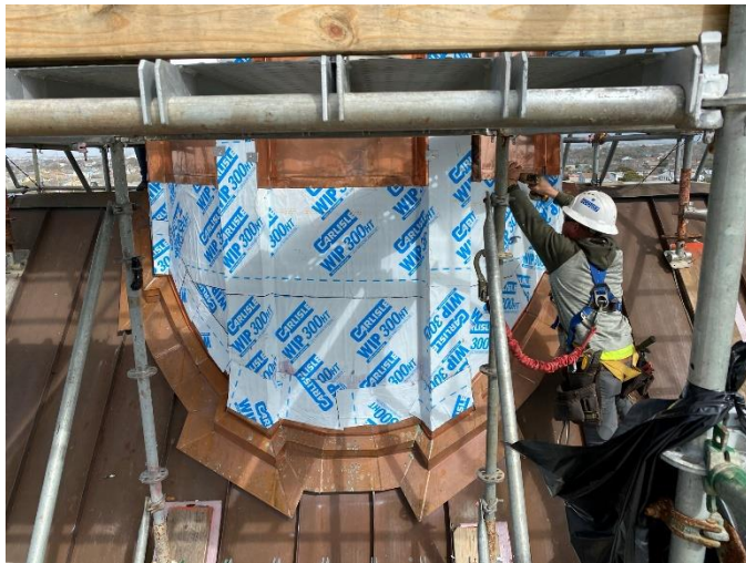
Photo11: Copper Cladding is Installed
