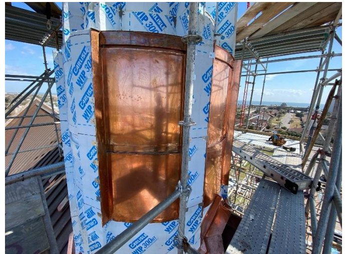
Photo04: Copper Cladding Installed with Clips
