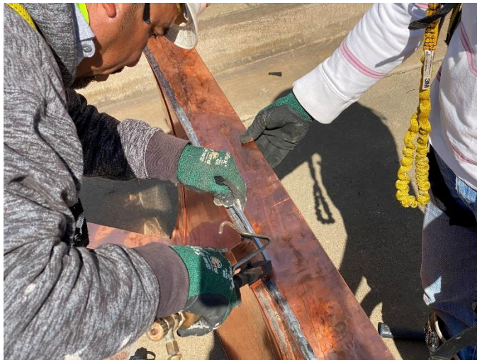
Photo03: Copper Joint is Soldered
