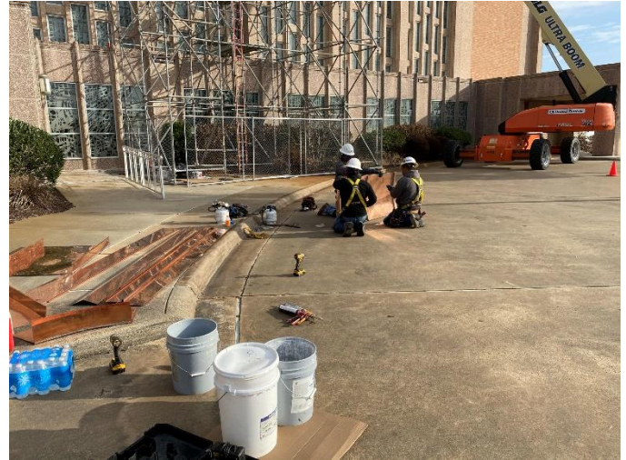
Photo10: New Copper Cladding Prepared for Installation
