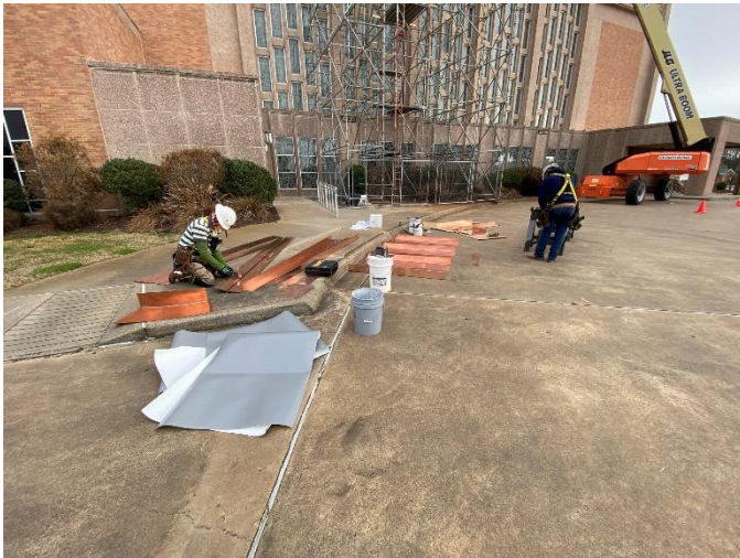
Photo15: New Copper Cladding Prepared for Installation
