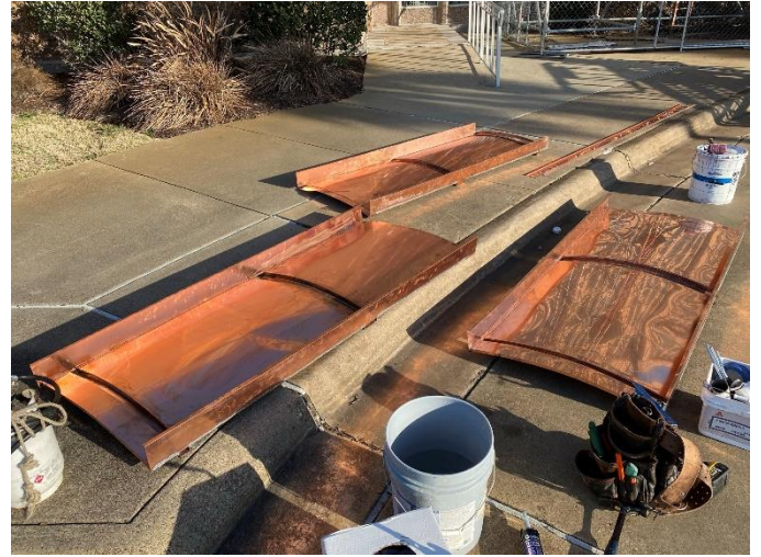
Photo06: New Copper Cladding Prepared for Installation
