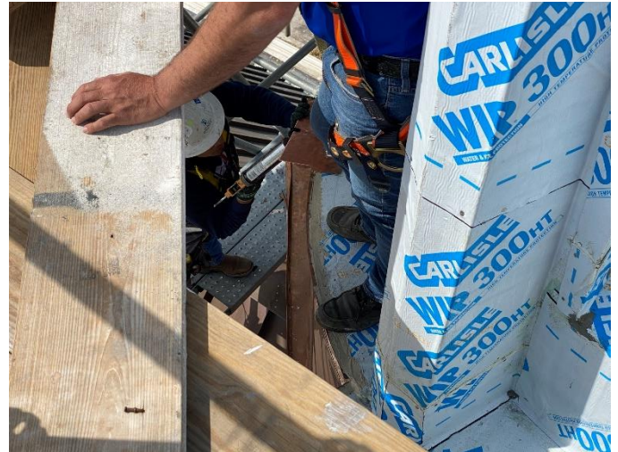
Photo22: Sealant Applied to Copper Joints
