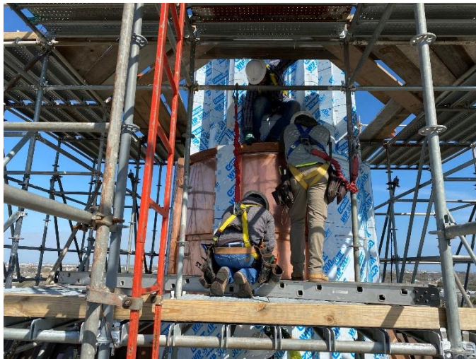
Photo07: Installation of Copper Cladding
