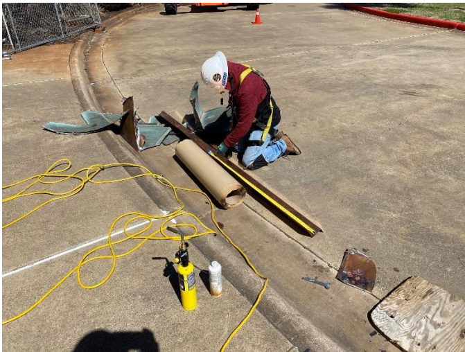
Photo11: Copper Flashing is Measured and Cut
