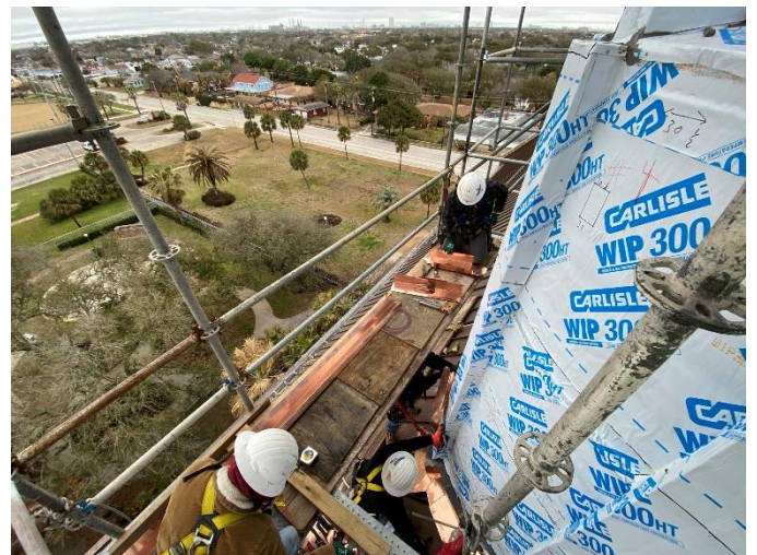
Photo08: Flashing is Installed
