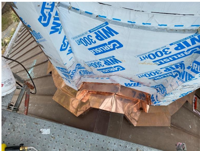
Photo21: Copper Flashing at Ridge of Roof Installed
