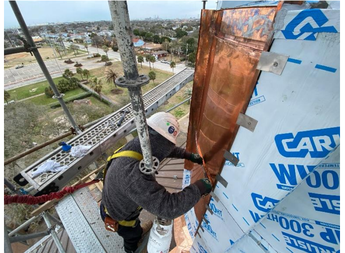
Photo24: New Cladding Installed
