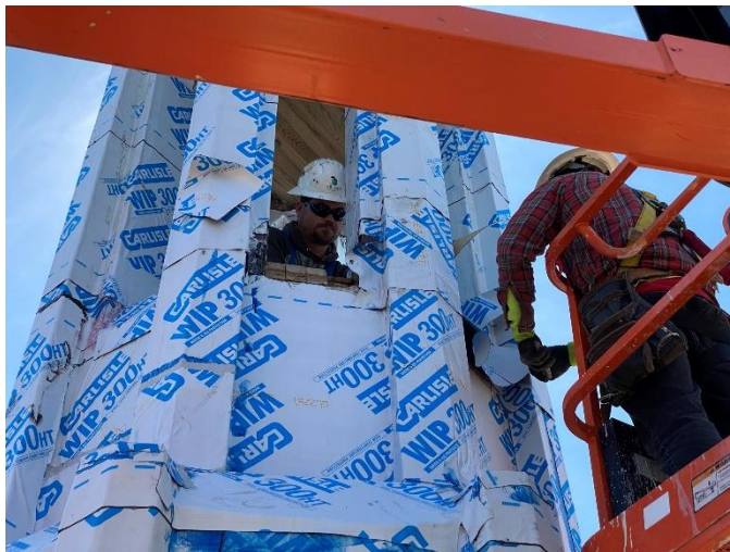
Photo17: Waterproof Membrane Details Around Steeple
