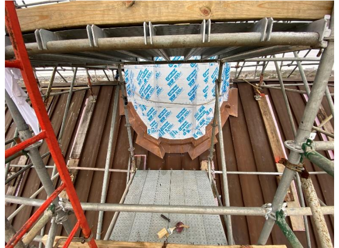
Photo06: South Side Base of Steeple Flashing Completed
