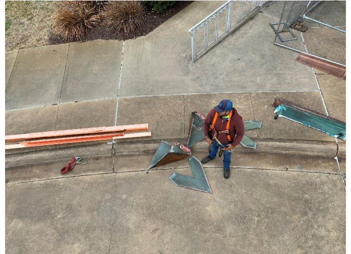
Photo02: Copper Pieces from Top Tier of Steeple on Ground
