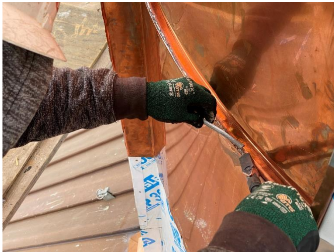
Photo25: Welded Joint Filed and Smoothed
