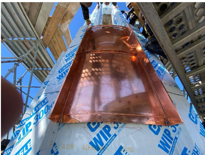
Photo13: New Copper Cladding is Installed
