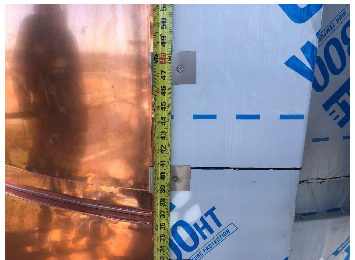
Photo14: Mounting Clips Spaced at Least 8" O.C.
