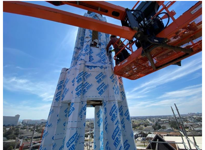
Photo16: Waterproof Membrane Details Around Steeple
