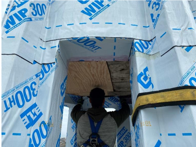
Photo23: New Wood Installed, Waterproofing Installed
