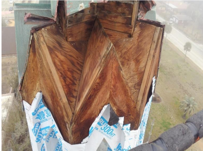
Photo01: Top Tier of Steeple is Stripped of Copper Cladding
