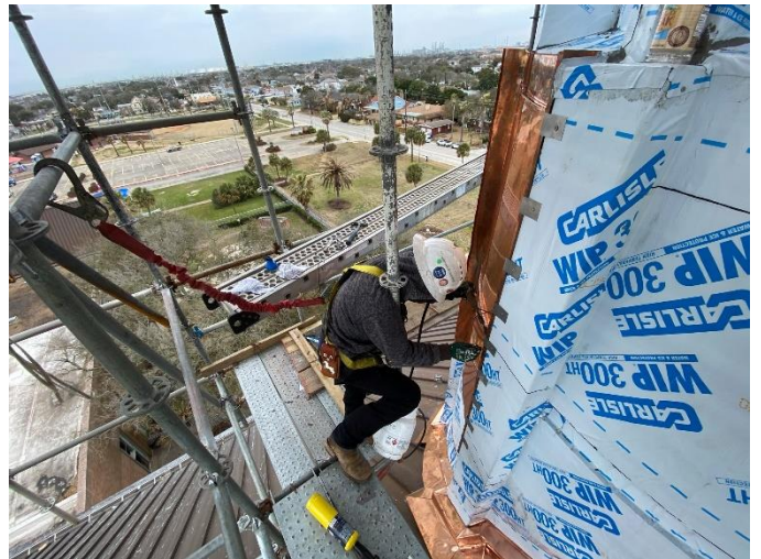
Photo26: Welded Joint Filed and Smoothed
