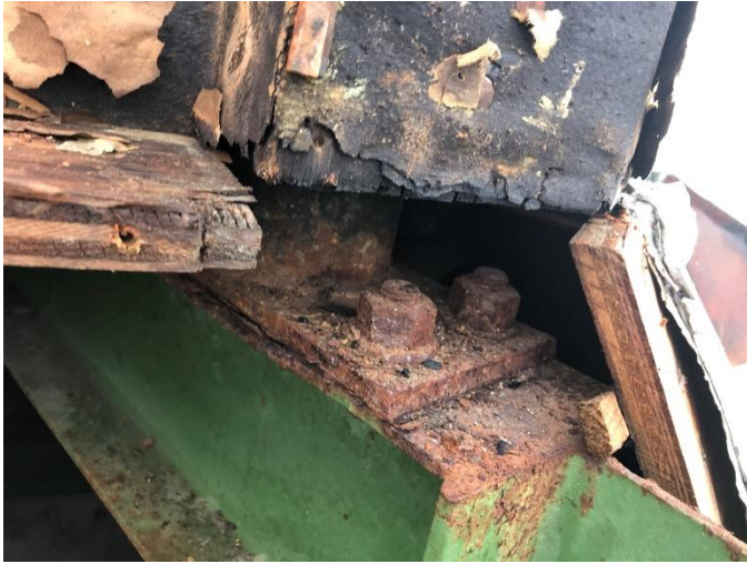
Photo13: Rusty Bolts Behind Copper and Wood
