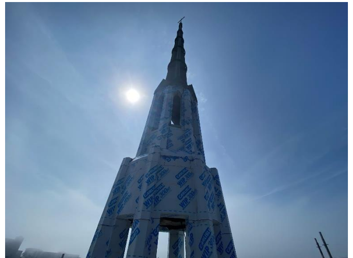
Photo26: Waterproof Membrane Reaching the Top Tier
