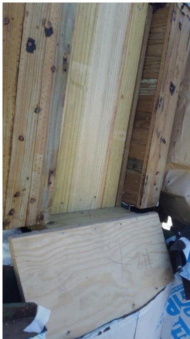
Photo08: 2x4s and Marine Grade Plywood Used to Repair Old Wood
