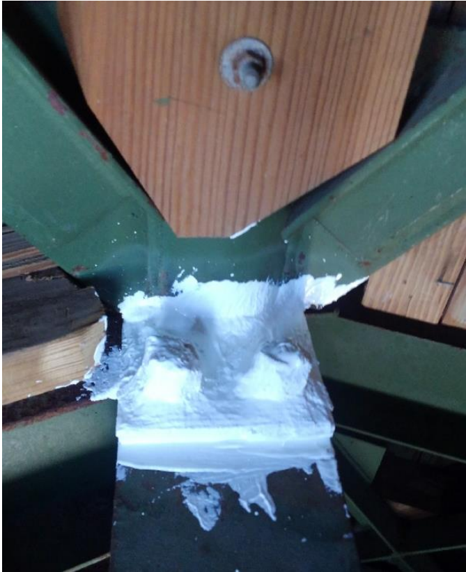
Photo17: PMMA Liquid Flashing Over Cleaned Bolts
