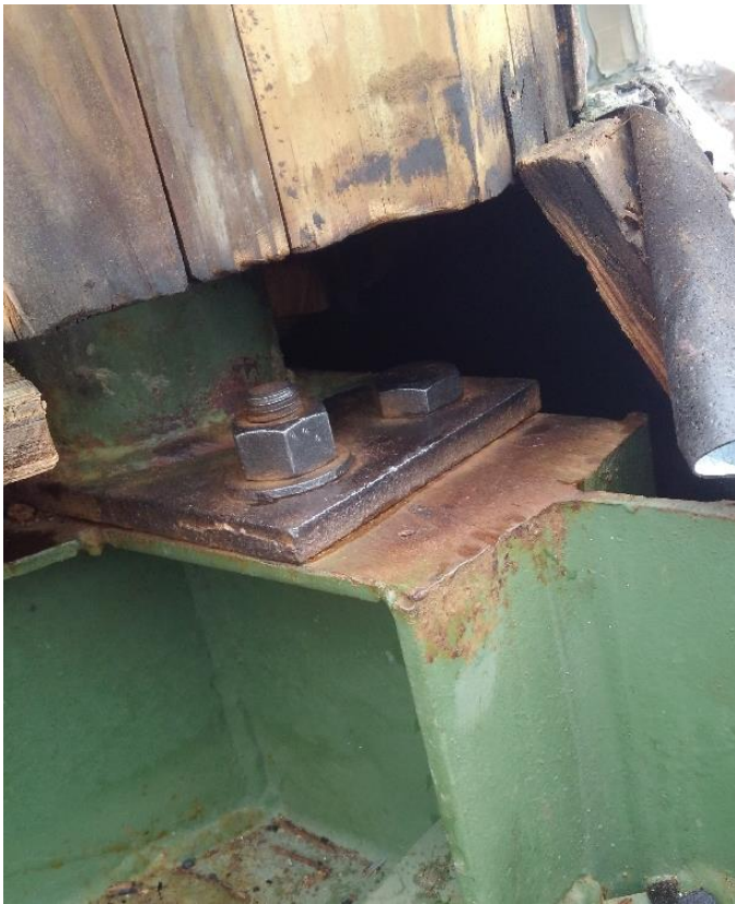
Photo15: Bolts and Beams are Cleaned
