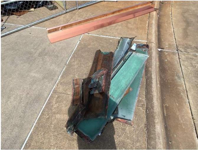
Photo23: Copper Cladding Removed
