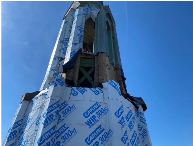
Photo03: Waterproof Membrane Applied to Next Tier
