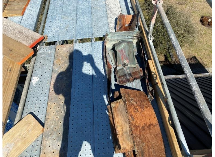
Photo02: Removed Copper Cladding
