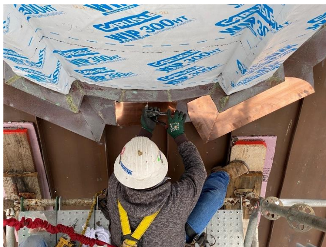
Photo12: Copper Flashing Installed
