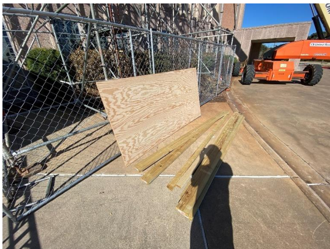
Photo05: 2x4s and Marine Grade Plywood for Repairs
