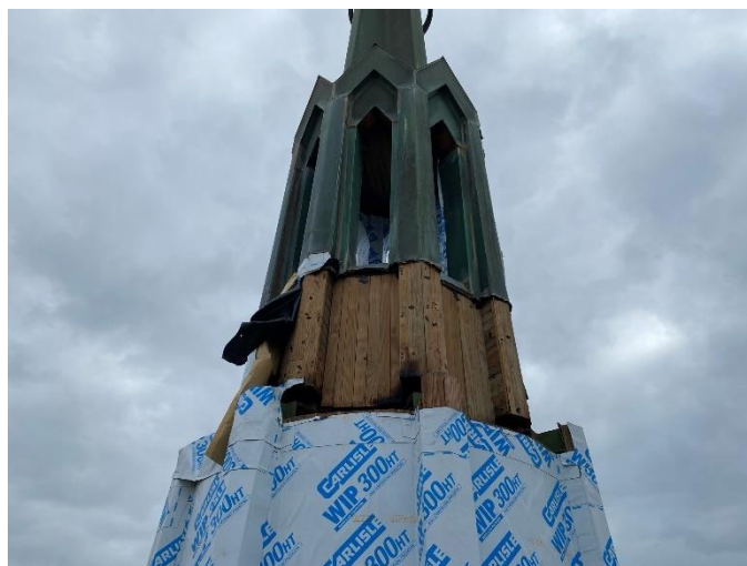
Photo10: Copper Cladding Removed from Upper Level of Steeple
