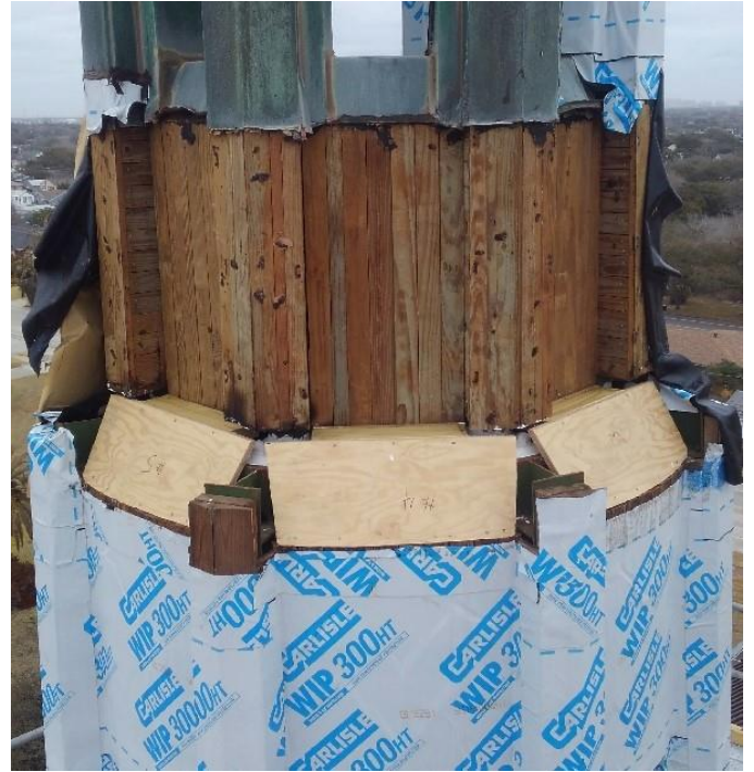
Photo20: Marine Grade Plywood Slants to Protect Steel Structure
