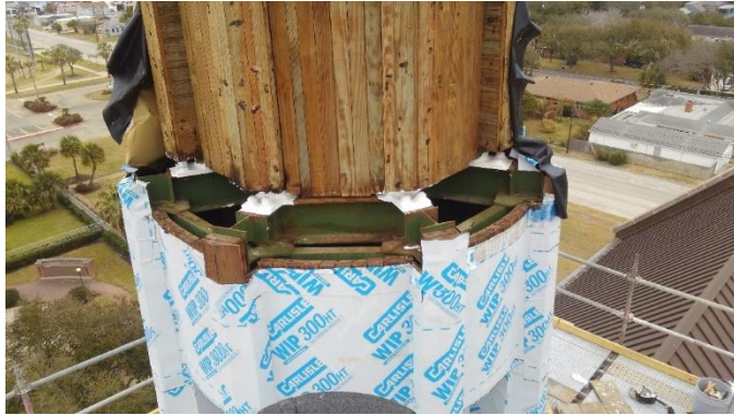
Photo19: All Bolts Cleaned and Coated with PMMA
