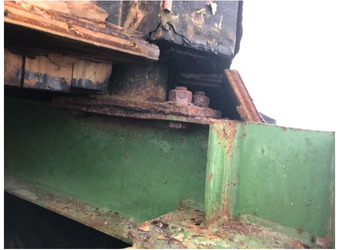
Photo14: Rusty Bolts Behind Copper and Wood
