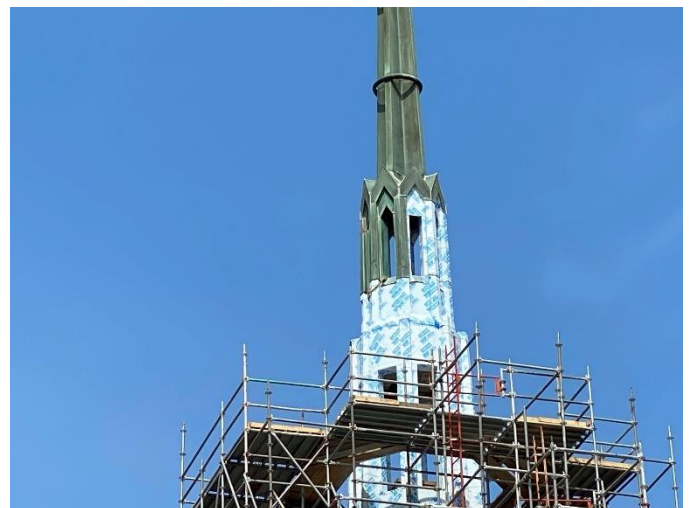
Photo22: Waterproofing Reaching the Top Tier
