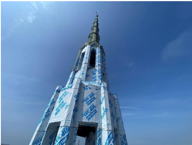
Photo25: Waterproof Membrane Reaching the Top Tier
