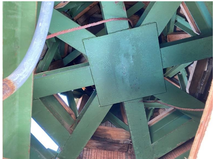
Photo04: Steel Structure of Steeple
