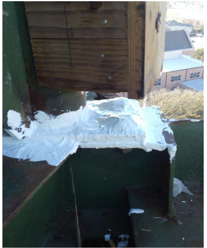
Photo16: PMMA Liquid Flashing Over Cleaned Bolts
