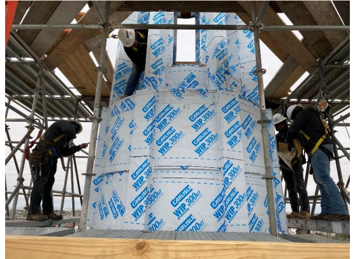
Photo23: Waterproof Membrane Applied Around Steeple
