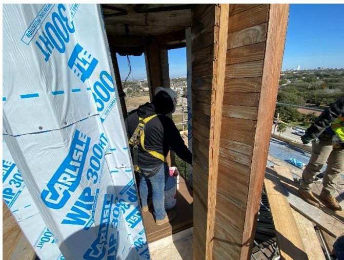
Photo09: Waterproofing Applied
