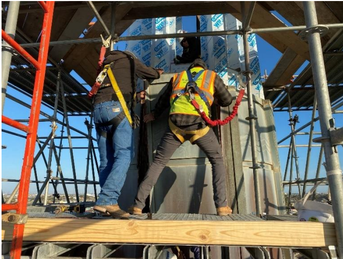
Photo11: Copper Cladding Removed from Base of Steeple
