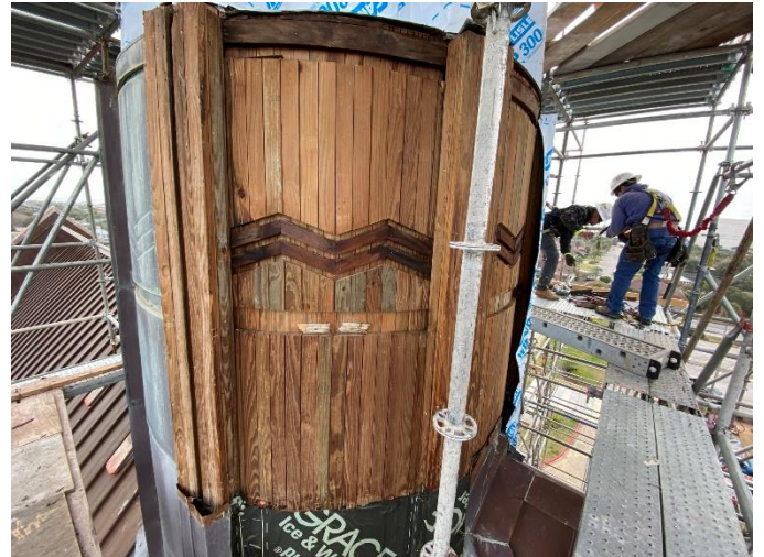
Photo16: Copper Cladding Removed at Base of Steeple
