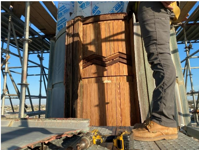
Photo13: Exposed Wood After Removing Copper
