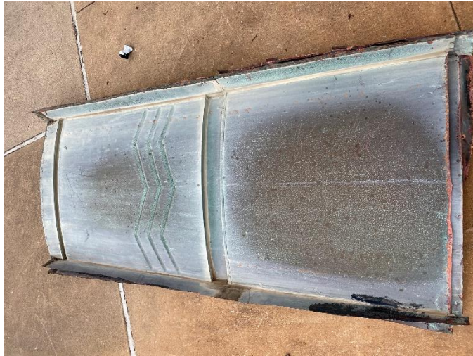
Photo22: Removed Copper Cladding
