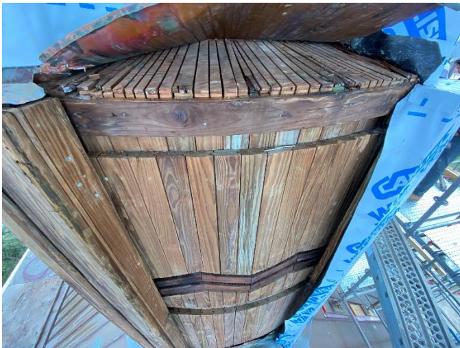
Photo17: Copper Top Removed from Base of Steeple
