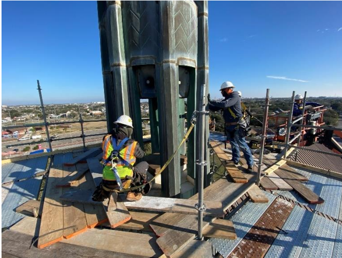
Photo01: RB Hash Begins Removing Copper Cladding
