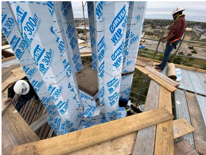
Photo24: Waterproof Membrane Applied
