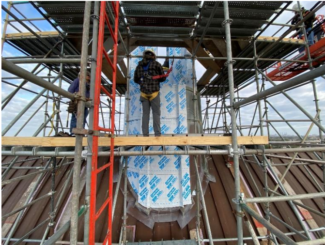
Photo15: Waterproof Membrane Applied
