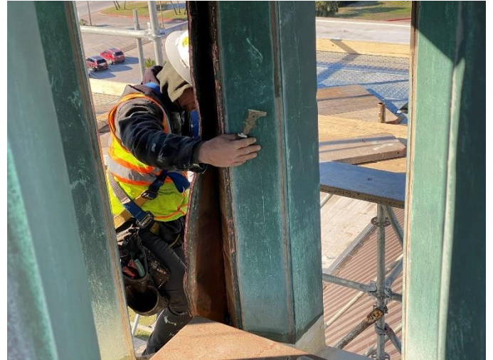
Photo02: Old Sealant is Scraped Away and Copper Removed
