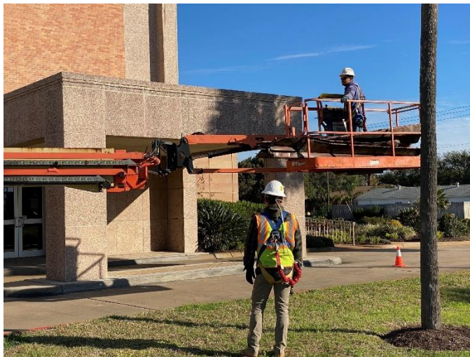
Photo07: Copper Cladding is Brought Down
