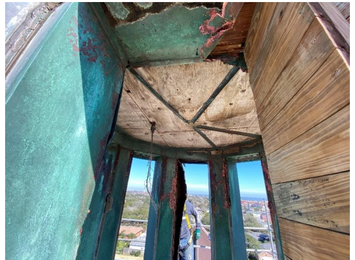
Photo04: Copper Cladding is Removed
