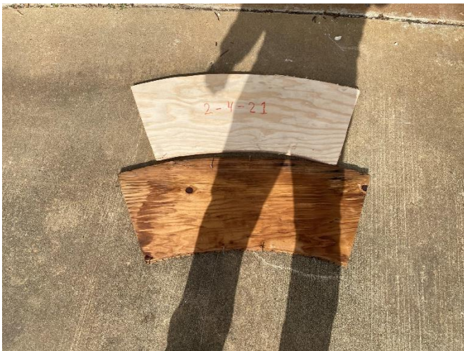
Photo21: New Wood is Cut to Replace Old Wood
