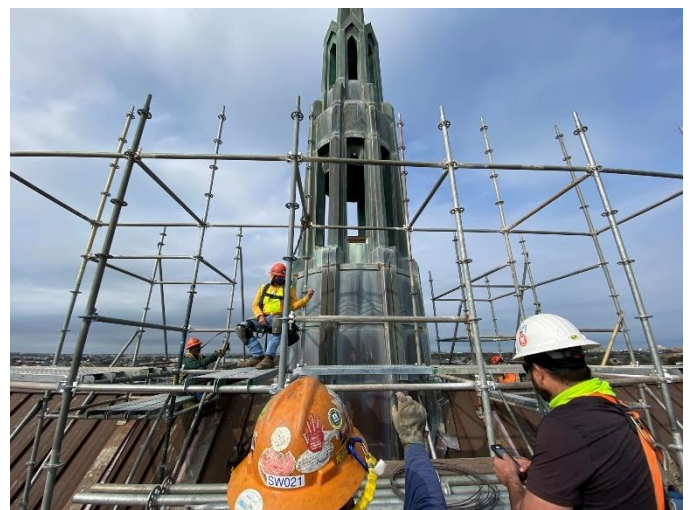
Photo04: Scaffolds Assembled Around Steeple
