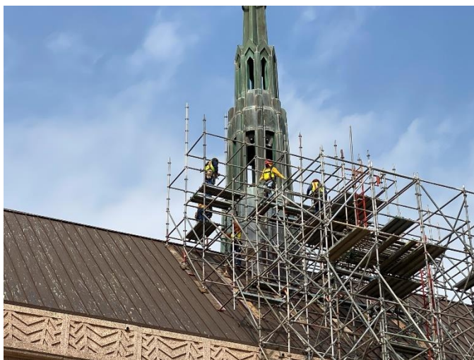
Photo03: Scaffolding Being Assembled
