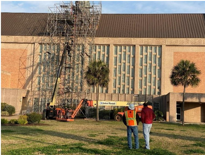
Photo05: Telescopic Boom Lift Brought on Site
