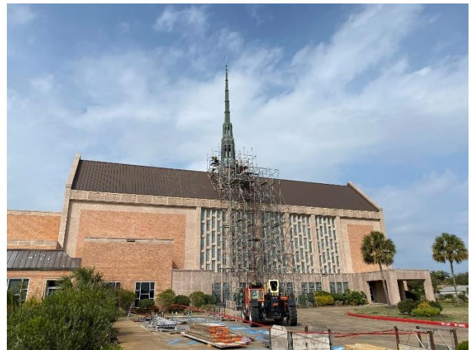
Photo02: Scaffolding Being Assembled
