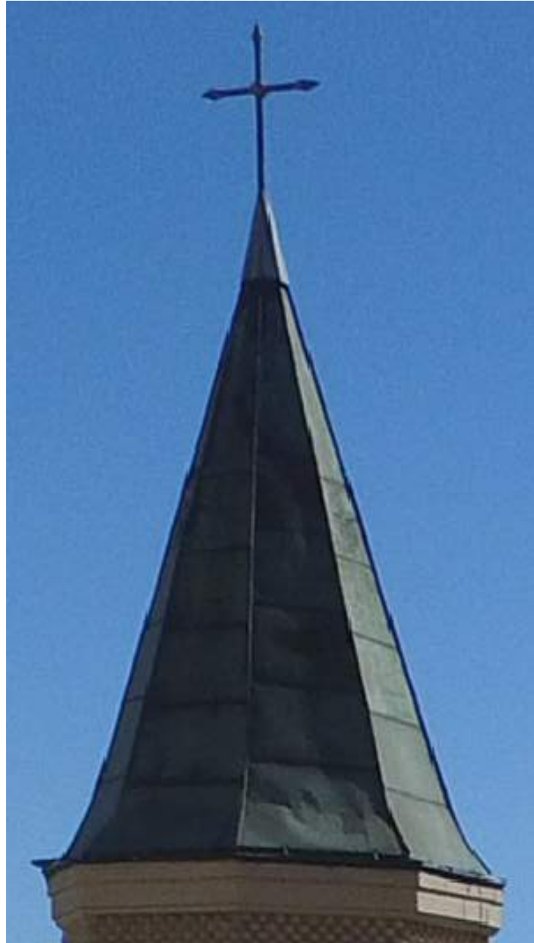
9 EXISTING SPIRE ROOF SCALE: N.T.S. (FOR REFERENCE ONLY)
